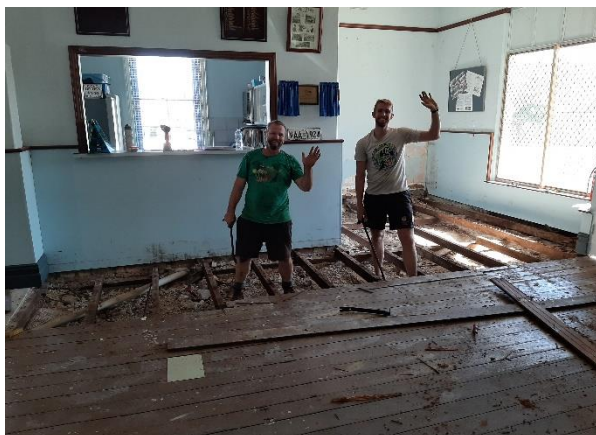
1 Jason and English George removing the wood floor
